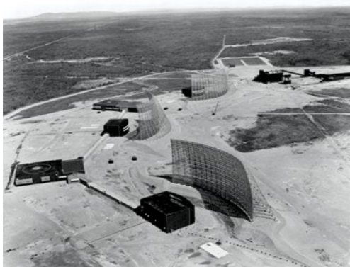
FIGURE 11: Example of a Ballistic Missile Early Warning System (BMEWS) radar station, part of a network to provide NORAD with early warning of incoming ICBM's. This station is BMEWS Site 2, near Anderson, Alaska, as seen in 1962
